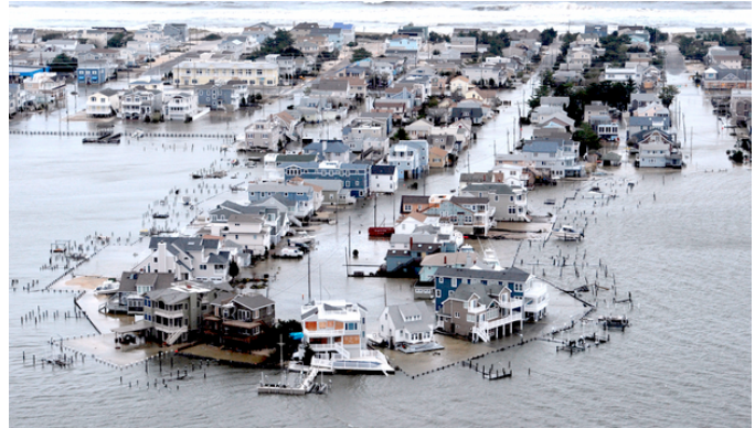
Portion of Long Beach Island, NJ after Hurricane Sandy
